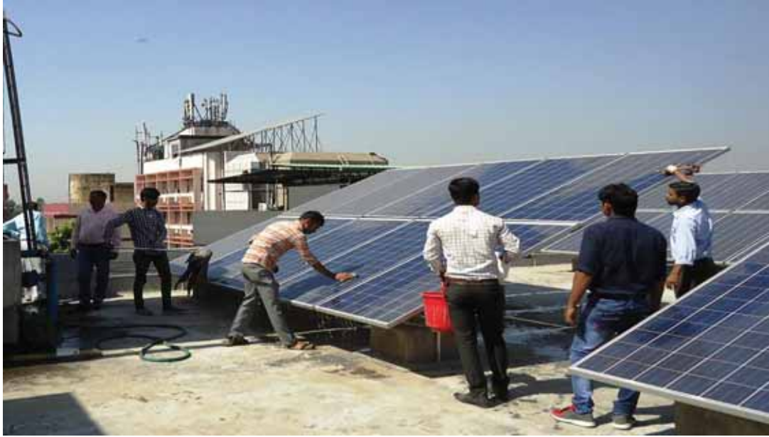
Cleanliness activities at Rooftop Solar plant
